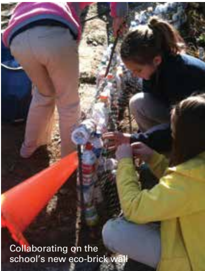
The foundation of Monarch's eco-brick fence
