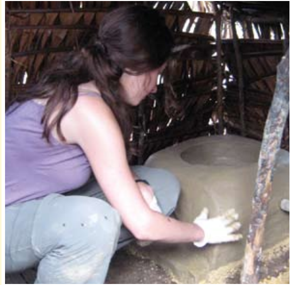
Smoothing the surface of an almost-done stove
